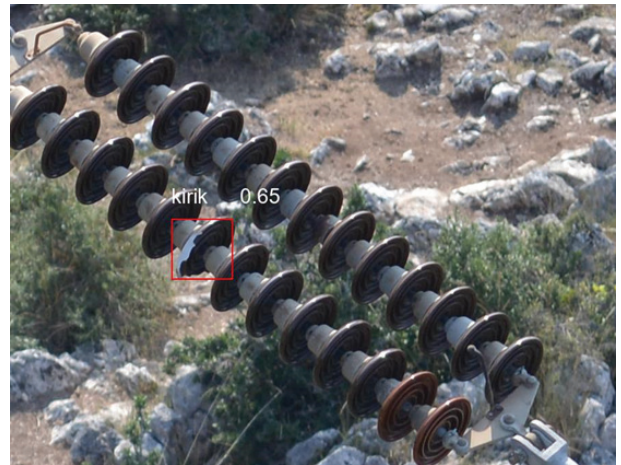
Figure 8: Detection of broken part fault on insulator
