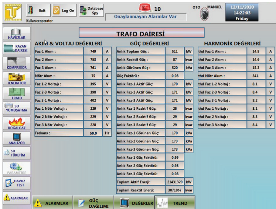
Figure 5. Substation Analyzer Data (Current, Voltage, Power Values)
