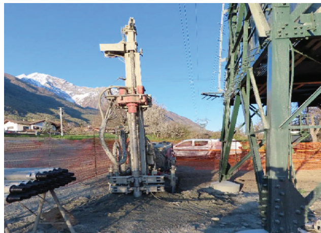
Figure 3. Installation of micropiles for the new grounding systems in the alps.
